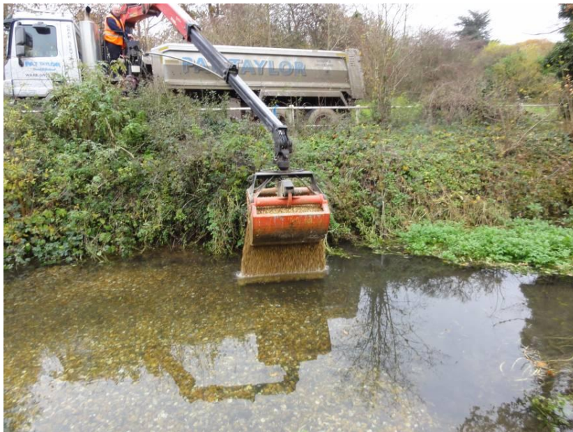
Replacing gravel n the River Mimram
